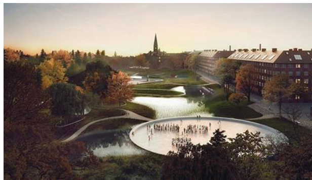
2. When completed, Copenhagen's Hans Tavsens Park will serve as a rainwater catchment for the inner “Nørrebro” neighborhood capable of capturing and delaying of 18,000 cubic meters of rainwater at any given time. (Courtesy of Dezeen)
